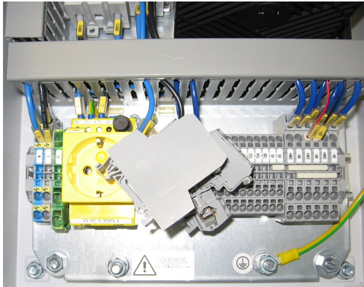
Figure 10 – Plastic Guard on Neutral Fuse Block
